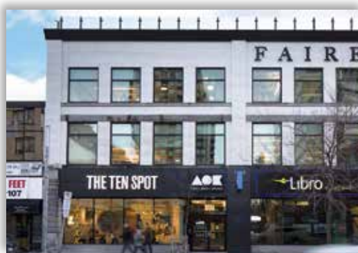
165 King Street, Kitchener (former Budd's Department Store)
