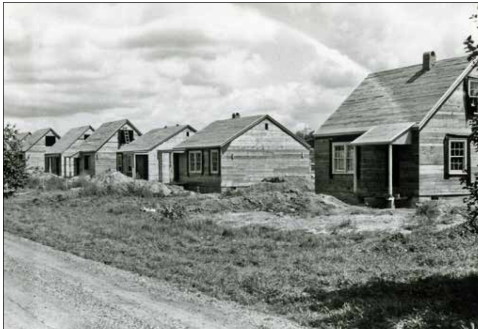
Wartime houses under construction in the east ward, mid-1940s. Photo courtesy of St. Marys Museum historic image collection.
