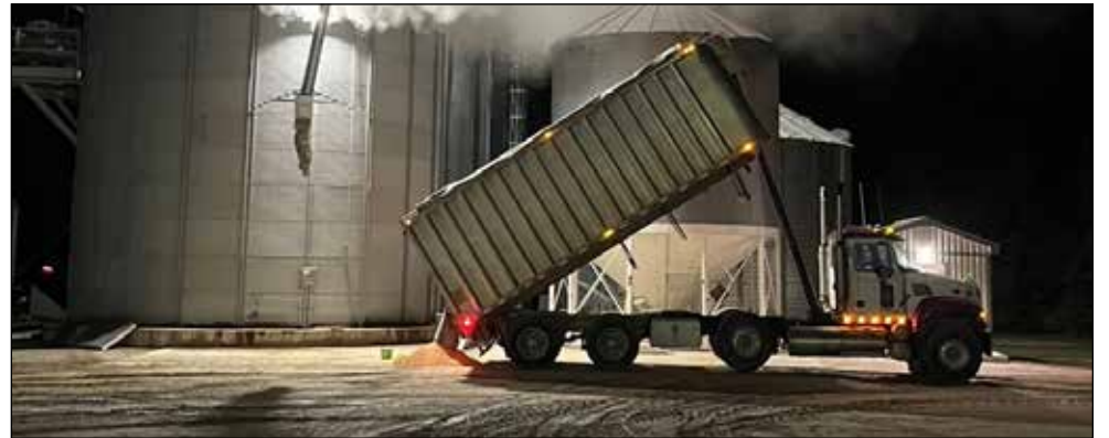
Even in the evening in darkness, unloading and drying continues at the Matt Drummond facility as the last corn is unloaded from this truck into the conveyor feeding the corn dryer.
