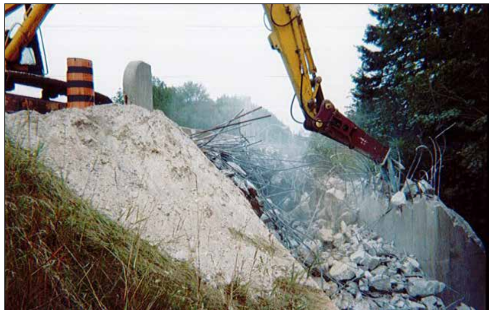
Above: The Blyth Tunnel being filled in.
