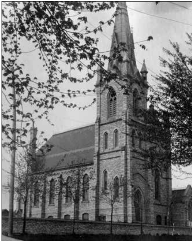
The Presbyterian Church, ca 1910. Except for some accessibility adaptations, this beautiful building looks the same today.
