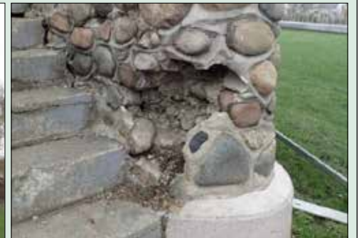
Left, Overall view of the gazebo structure. Above, Mortar deterioration and stone loss at step sidewall location (Source: RIMKUS Structural Review of Gazebo, dated April 27, 2023)
