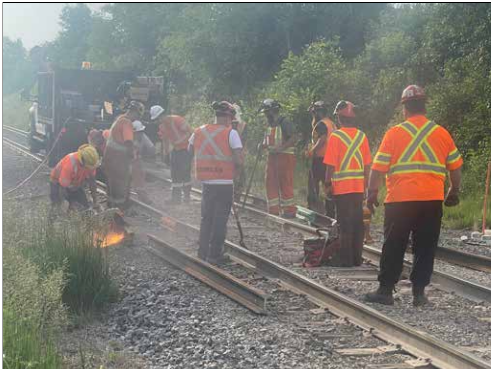
CN workers replacing a railway track between Shakespeare and New Hamburg. (Photo credit: Gary West)
