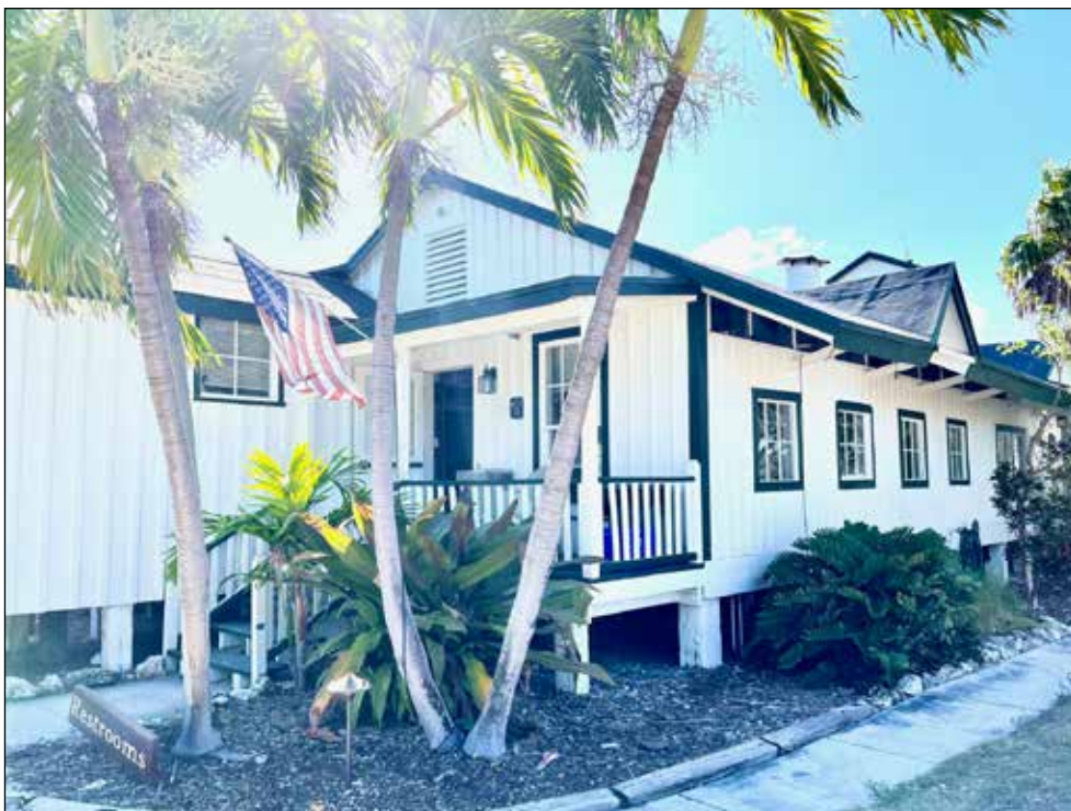
One of the buildings that remain from the railroad work camp that housed 400 men on this tiny island.
