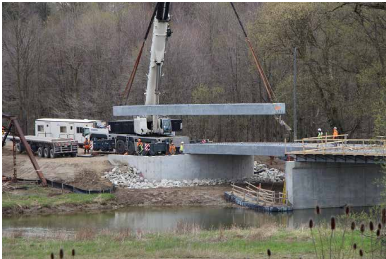
Construction workers placing short girders on the east side of the Bridge Street bridge reconstruction project. The project was awarded to Sierra Bridge of Woodstock in June 2022 for $4.8-million. (Photo credit: Anne Loeffler)
