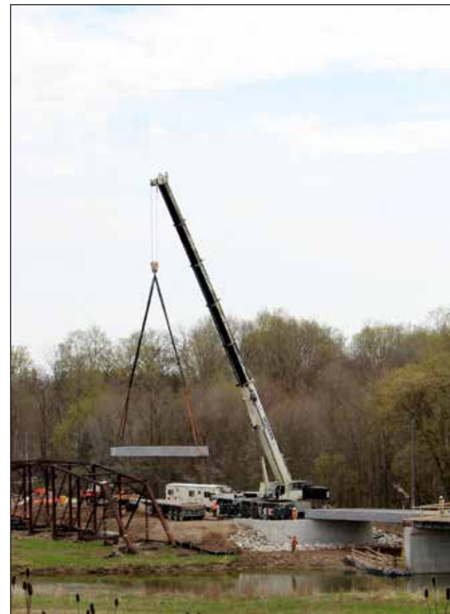
Construction workers placing short girders on the east side of the Bridge Street bridge reconstruction project. The project was awarded to Sierra Bridge of Woodstock in June 2022 for $4.8-million. (Photo credit: Anne Loeffler)
