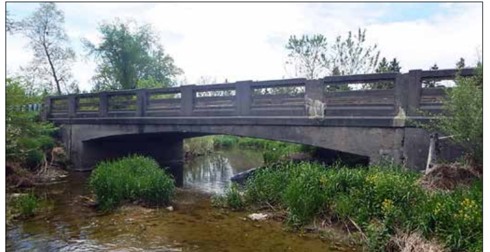
The Dewar Bridge.
