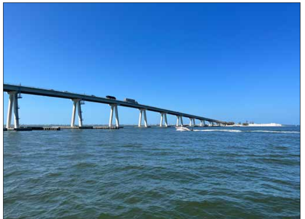
The bridge from Fort Myers to Sanibel Island was breached in five places by Hurricane Ivan. But it was repaired and re-opened within a month.
