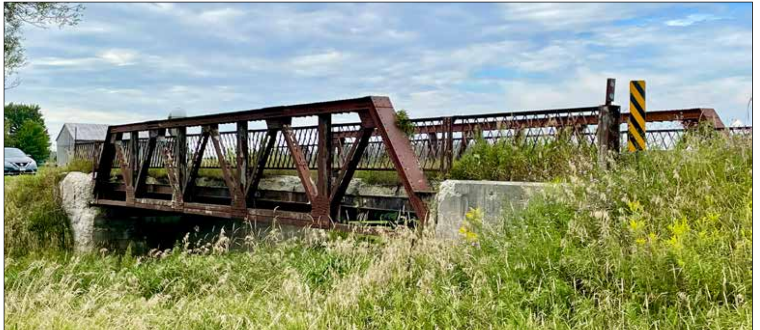
The old Warren pony truss bridge across Whirl Creek.
