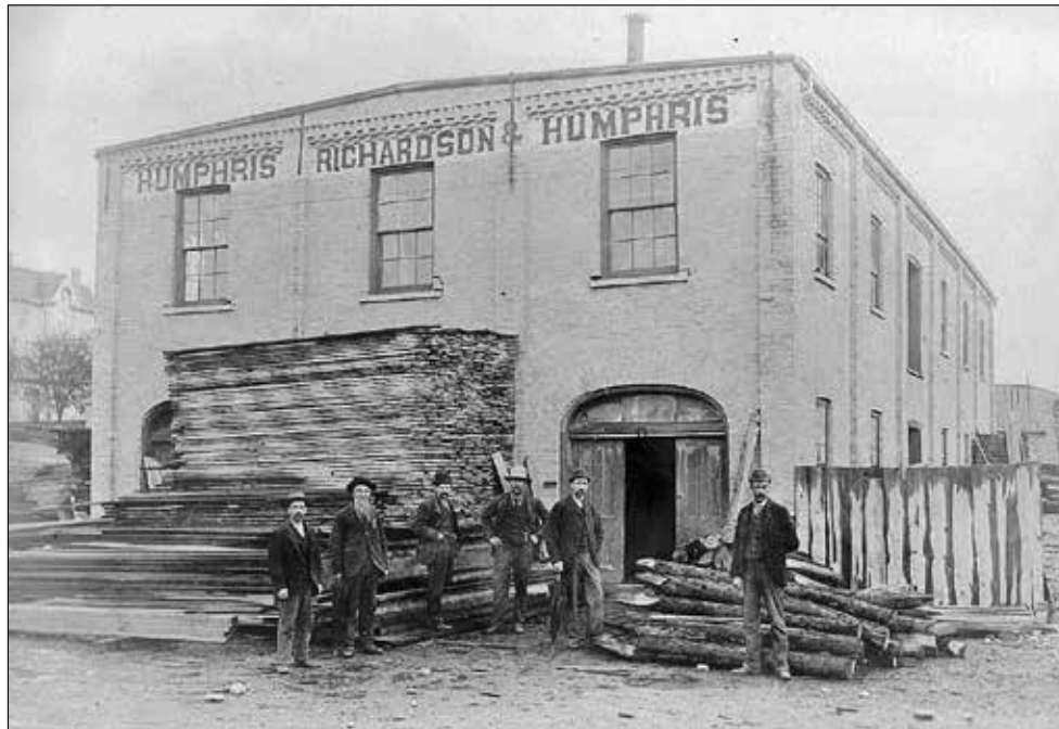
The owners and workers stand in front of the west façade of the Humphris, Richardson & Humphris Planing Mill. J. A. Humphris is second from the right. Today, this building is O'Leary's Bar and Grill.
