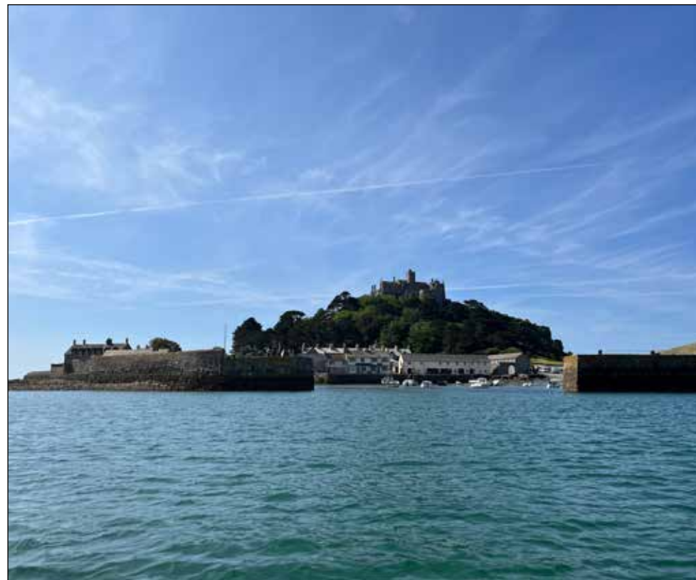
The view when approaching St. Michael's Mount by boat, at high tide.
