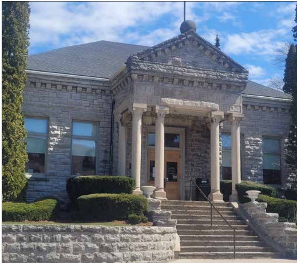
A disagreement over library services funding this year has left Perth South residents without access to books and other materials from the St. Marys Public Library Photo by Wendy Lamond
