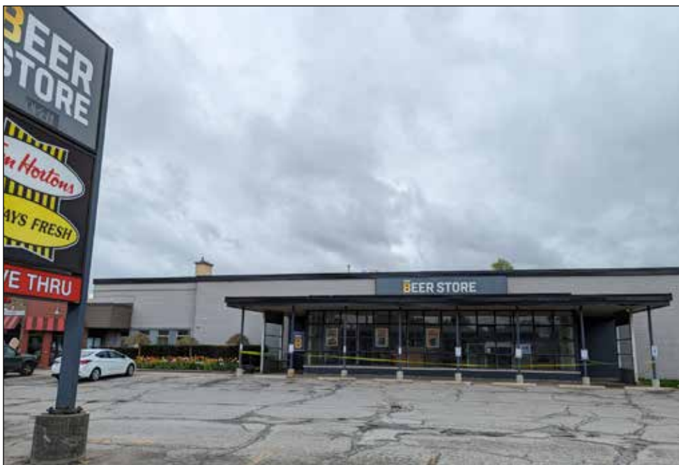
The Beer Store on Huron Street in Stratford remains closed as the investigation into an overnight fire May 6, which Stratford police has deemed suspicious, continues.
