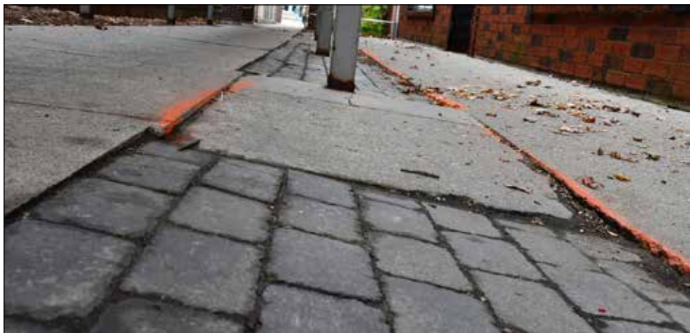
The unevenness between the bricks and sidewalk in front of One Library Lane is a hazard and creates an accessibility challenge, business owners allege. (JEFF HELSDON PHOTO)
