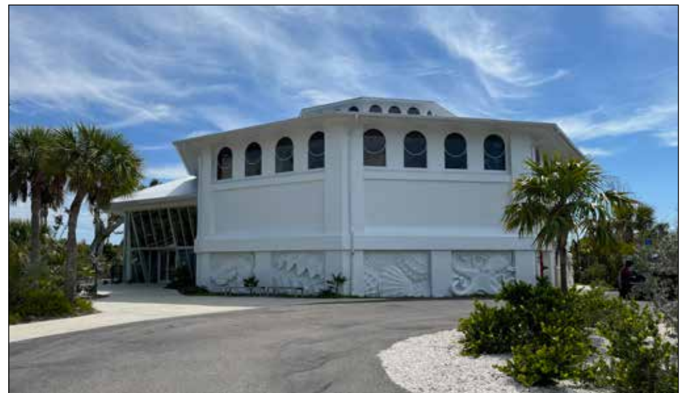
The Bailey-Matthews Shell Museum and Aquarium on Sanibel Island, now reopened after being severely damaged by Hurricane Ian.
