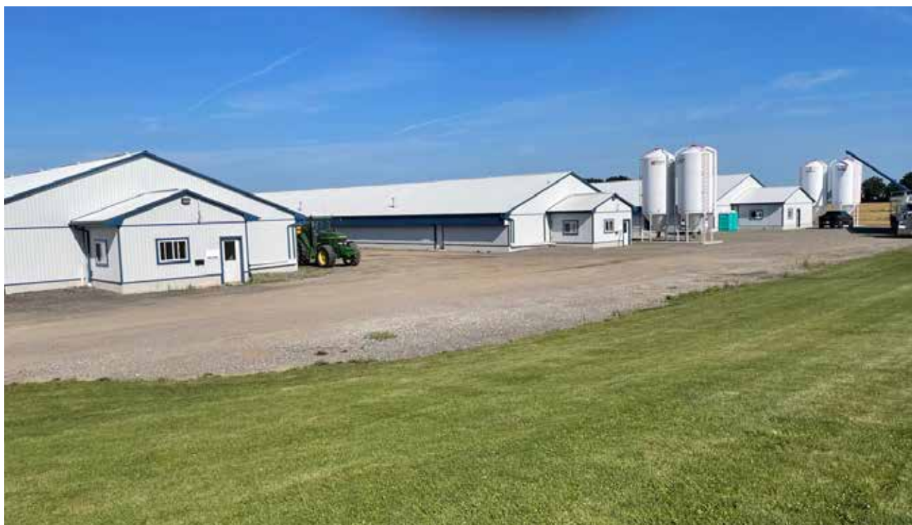
Talbot Road Poultry’s three barns use an all-in-all-out system to grow 50,000 broilers each time.
