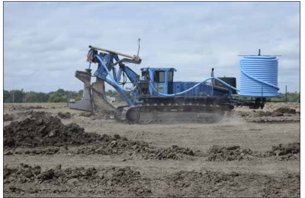
Visitors watch a demonstration of how drainage systems get installed. ~ Luke Edwards photos
