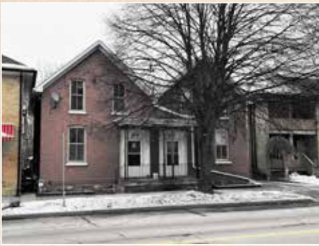
179-181 Peel Street, home of Joseph Umbach, 1904-1910
