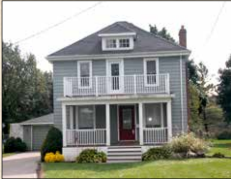
299 Bleams Court, built by Joseph Umbach in 1871
