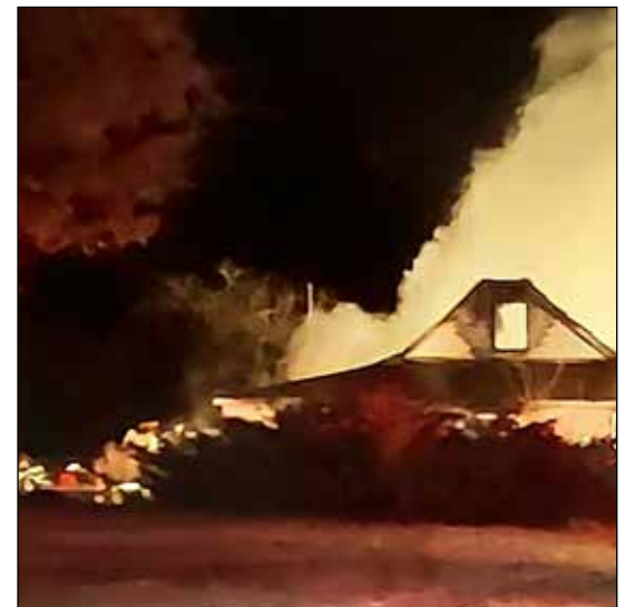
An abandoned house on Concession 6 Townsend between Angling Road & Old Highway 24 is in flames, Jan. 21, reported about 11:30 p.m. OPP
