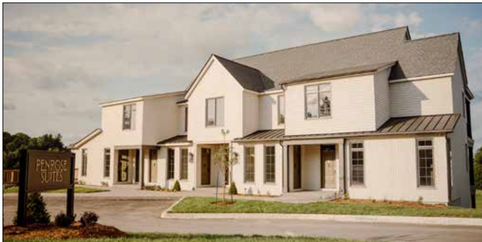
Phase I of the Penrose Suites opened for business in the summer of 2024. Contributed photo
