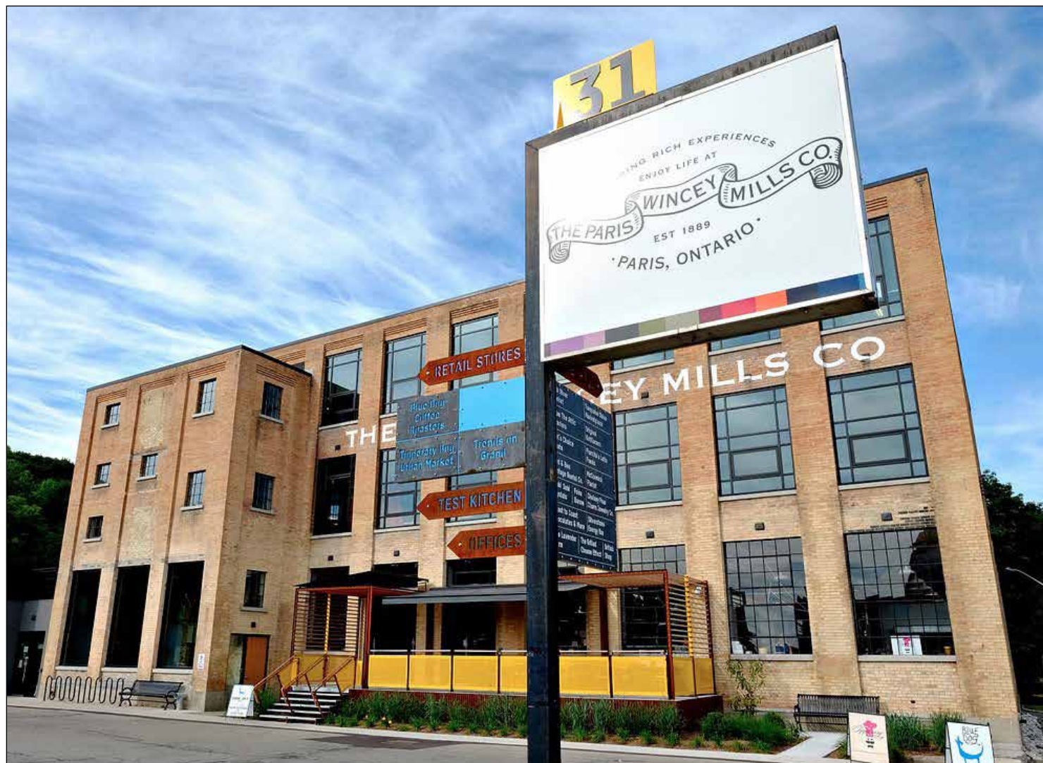
Located in Downtown Paris, The Paris Wincey Mills Co. is a historic building that dates back to 1889.
