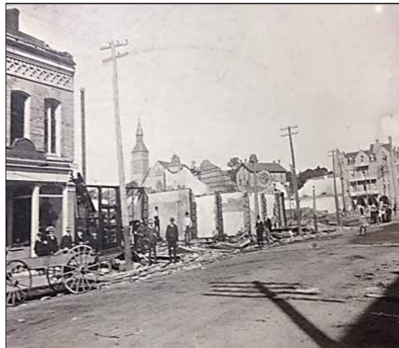
This photograph shows the West Side of Grand River St. North downtown Paris after the Great Fire of 1900. The town would quickly rebuild starting with a magnificent new Federal Post Office building on the site of the Roller Mills where the fire first started.
