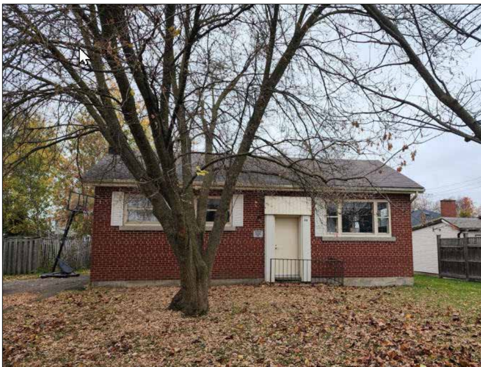
246 Railway Ave. is one of the properties investStratford hopes to activate as affordable or attainable housing.
