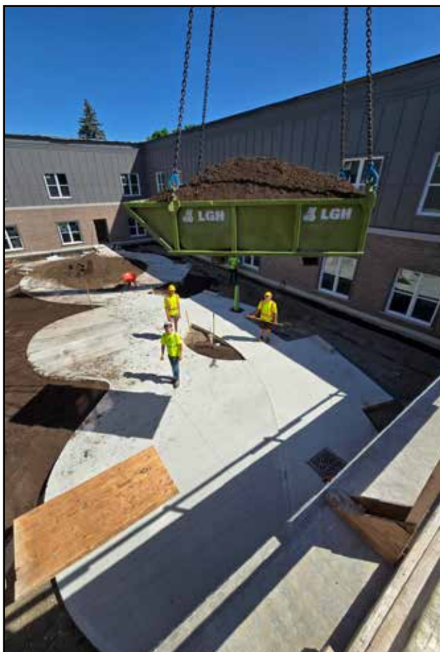
peopleCare's new Tavistock home recently had its outdoor courtyard filled with topsoil. The dirt was brought in via a large steel bucket hooked up to a crane. Contributed photo
