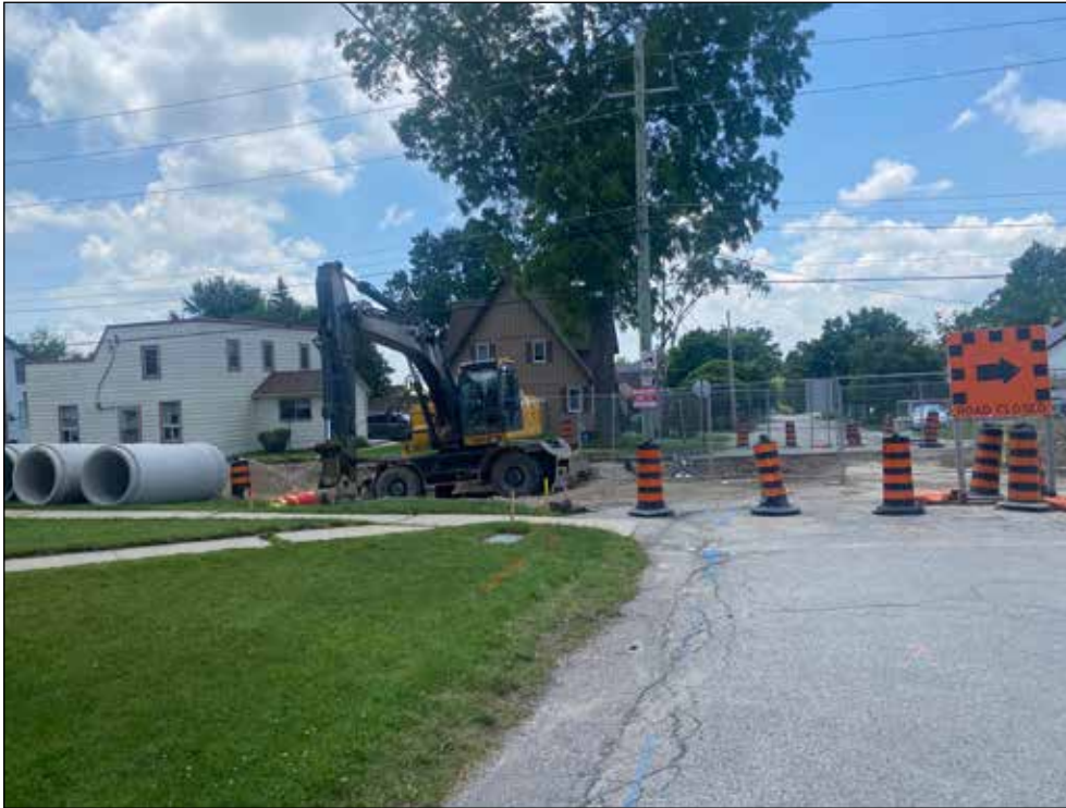
The progress on the Queen's Bush Road construction taking place in Wellesley village as of Sunday, June 25. The reconstruction is being undertaken by Kieswetter Excavating for about $2.1 million. This phase of the project will involve the replacement of all storm water infrastructure, replacement of curbs and sidewalks and base course asphalt. The full project will take place over three years. (Photo credit: Veronica Reiner)
