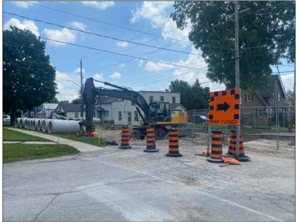
The progress on the Queen's Bush Road construction taking place in Wellesley village as of Sunday, June 25. The reconstruction is being undertaken by Kieswetter Excavating for about $2.1 million. This phase of the project will involve the replacement of all storm water infrastructure, replacement of curbs and sidewalks and base course asphalt. The full project will take place over three years. (Photo credit: Veronica Reiner)
